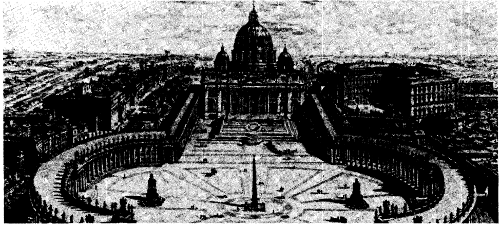
St. Peter's, with Forecourt and Colonnades. Bird's-eye view. 120, 1
