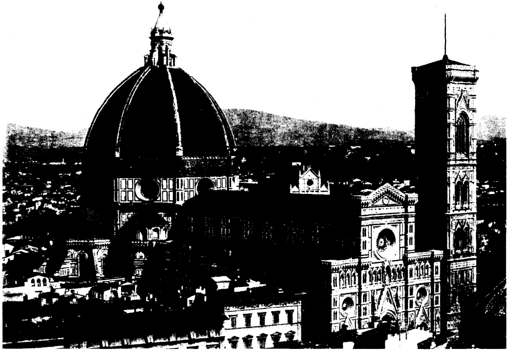
Cathedral and Campanile, Florence, Italy.
