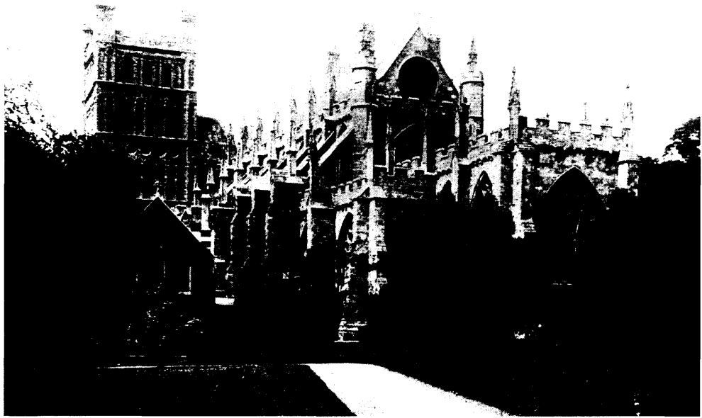
East End. Cathedral, Exeter Mainly Gothic. 1270—1369. Towers Norman. XII Cent.
