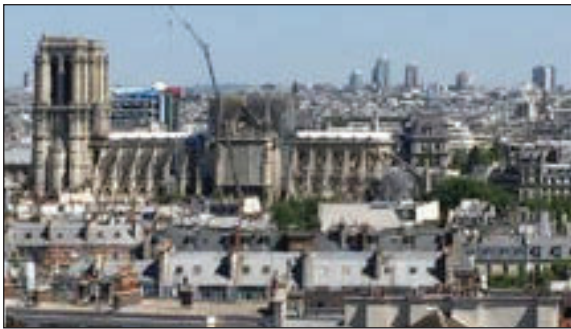
View of the work on Notre-Dame Cathedral from the terrace of Maurice Duruflé's apartment.
